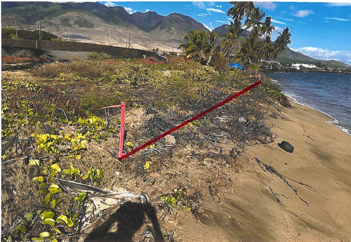
PICTURE # 2: SHORELINE TMK (2) 4-5-004:047 AT 5:00 PM ON AUG. 21, 2025.
