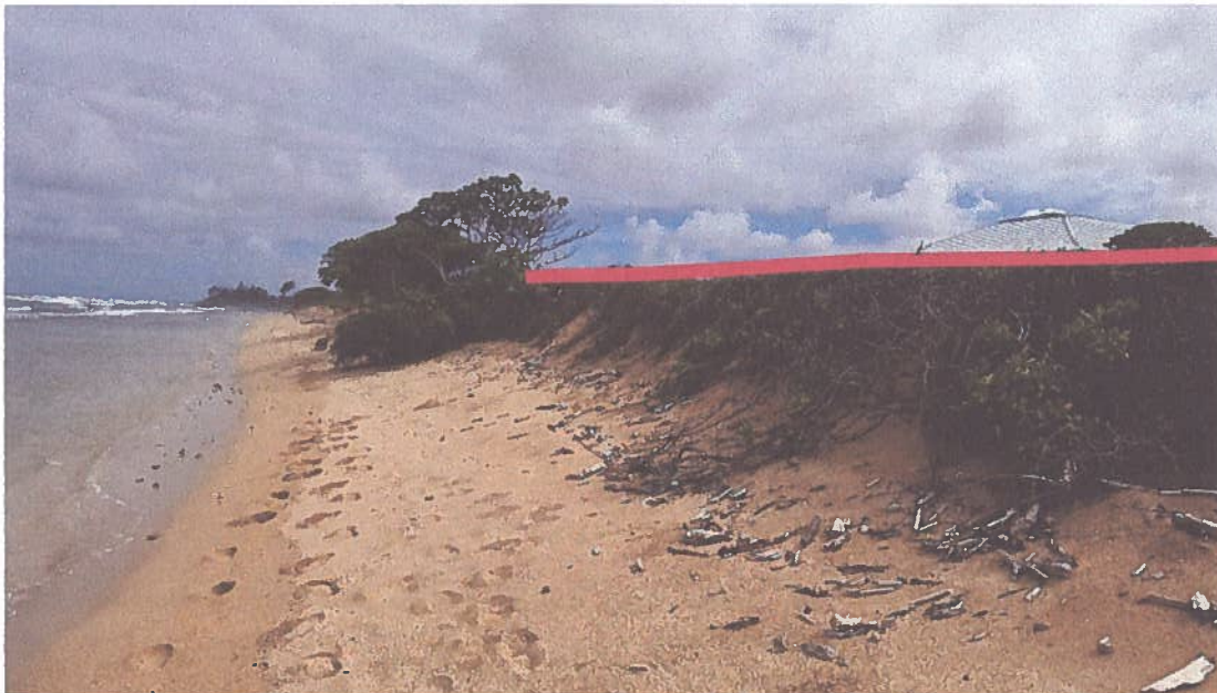
Picture 2: Facing Southwest
