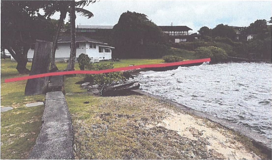
Picture 3: Facing northwest
