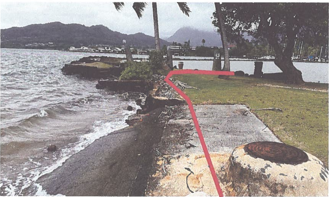
Picture 4: Facing southwest
