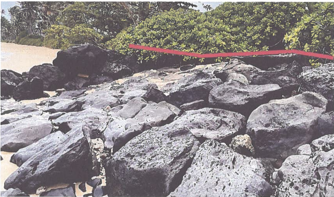
Picture 2: Facing Southwest
