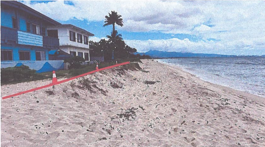
Picture 1: Facing East
