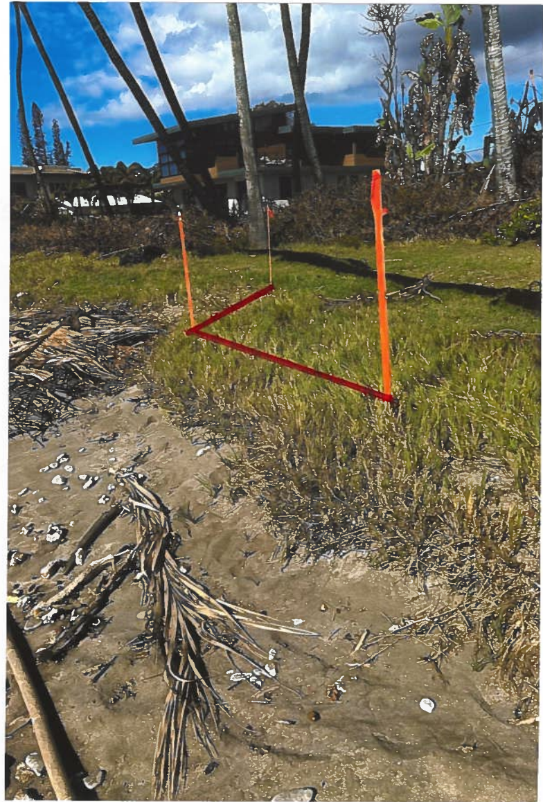
PICTURE # 6: SHORELINE TMK: (2) 4-6-002:002 AT 2:00 PM ON FEB. 29, 2024.
