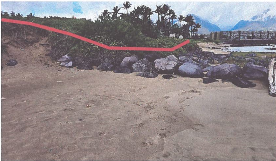
Picture 4: Facing Southwest
