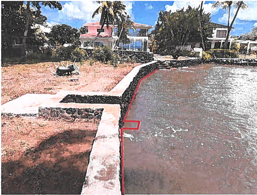
Photo No. 2 – September 8, 2022 – 2 P.M.
