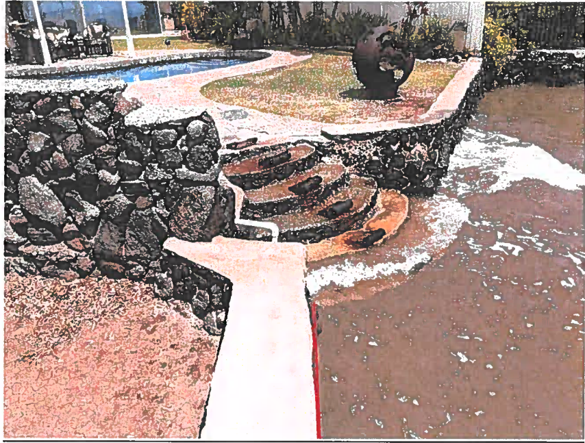
Photo No. 3 – September 8, 2022 – 2 P.M.
