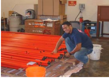
Casey Daniel of Heide & Cook prepares fire sprinkler pipes for installation
