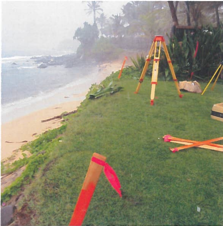
PHOTO 2 TMK:(2)2-6-12:31 SEPTEMBER 13, 2016 @ 11:30 A.M. & OCTOBER 20, 2016 @ 8:30 A.M.
