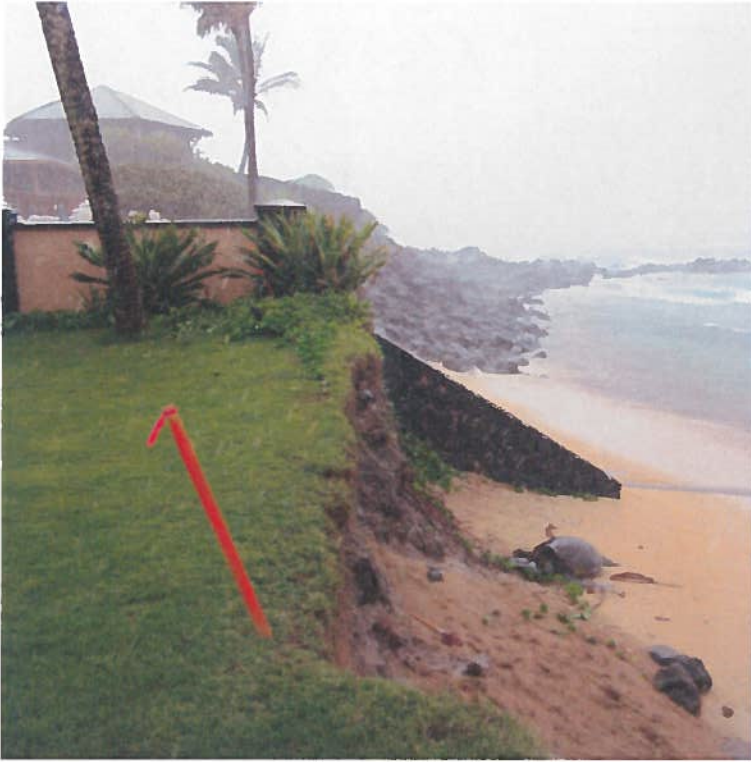
PHOTO 1 TMK:(2)2-6-12:31 SEPTEMBER 13, 2016 @ 11:30 A.M. & OCTOBER 20, 2016 @ 8:30 A.M.
