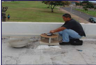
Jesse Raboy repairing ventilation fan unit at Maui High School
