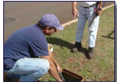
Dennis Silva replacing hose bibb at Kapa'a Middle School
