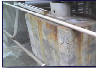
Cracked pedestal for the cooling tower at the Ke'elikōlani Building
