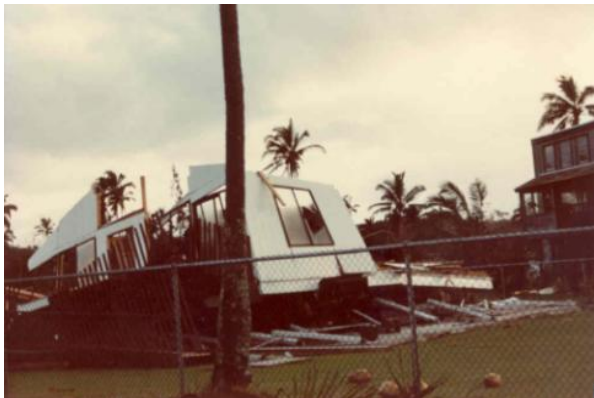
Example of severe hurricane damage to a home: loss of roof sheathing and roof framing structure, windows breached by windborne debris, and failure of wood foundation posts and beams.
